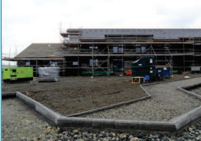
Mull Progressive Care Centre under construction
